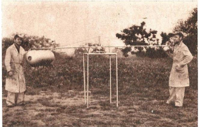
This working model of the all-metal vacuum dirigible runs on a counter-balance shaft which permits it to move in any direction.
