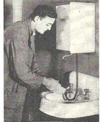
Hot water is instantly available anywhere in the house by means of a portable electric heater which holds two gallons. It can be attached to the faucet by a copper or rubber hose.
