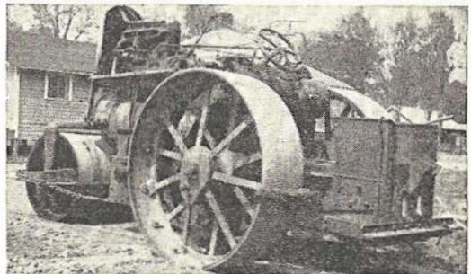
This is a steamroller that is no longer a steamroller! William Press converted it into a gasoline powered roller, using a 1930 Buick engine for the purpose. It will work an eight-hour day on only seven gallons of gasoline.
