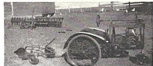
Marvin Green constructed this plow and tractor from odds and ends he collected on his farm. The tractor is powered with a 3/4 horse power engine. A governor holds its speed down to three miles an hour, so Marvin's five-year-old son can drive it.
